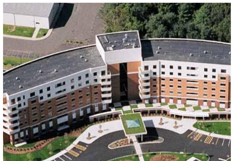
The "green" roofs at the porte cochere and "Main Street" rooftop help support the Owner's sustainability goals.
