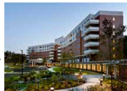
The balconies represented a significant design challenge, both in terms of constructability and long-term maintenance requirements.
